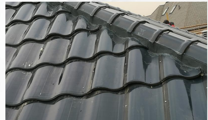
North slope open mold and close edge tiles
